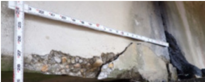
Figure 6: Concrete Spall/Delamination at Beam 2-6
