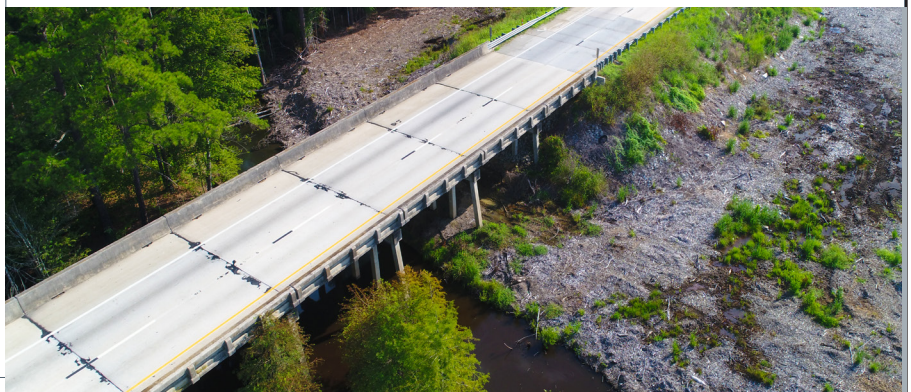
Figure 2: Expansion Joints in Need of Repair
