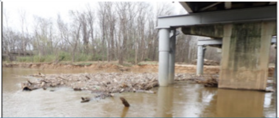
Figure 3: East Face, Crutch Bent with Timber Debris Buildup
