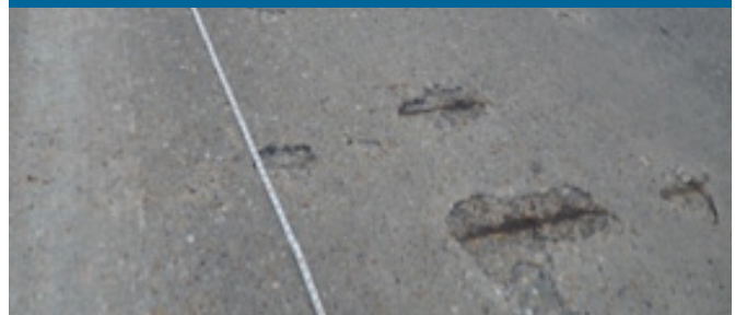
Figure 9: Concrete Spall/Delamination on Roadway Deck w/ Exposed Rebar at Span 3
