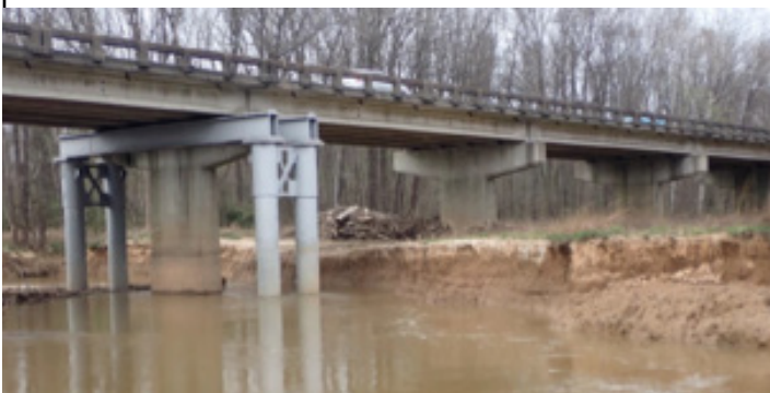
Figure 15: East Embankment, Crutch Bent with Eroding Bank in Background
