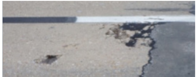
Figure 7: Concrete Spall/Delamination on Roadway Deck at Span 1
