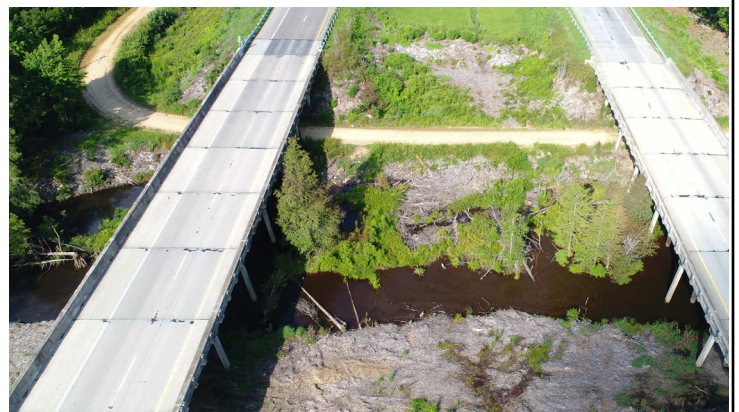
Figure 16: Timber Debris Eroding into Channel
